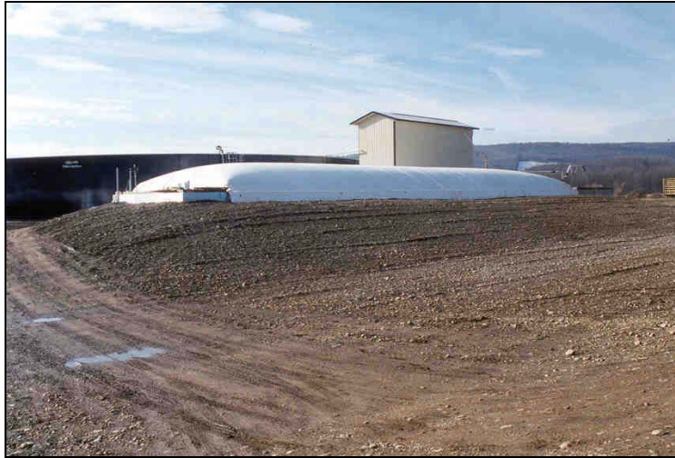
Figure 4. Plug Flow AD System
