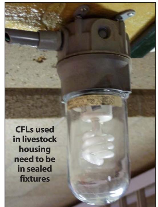
**Figure 8. Energy efficient lights.**
