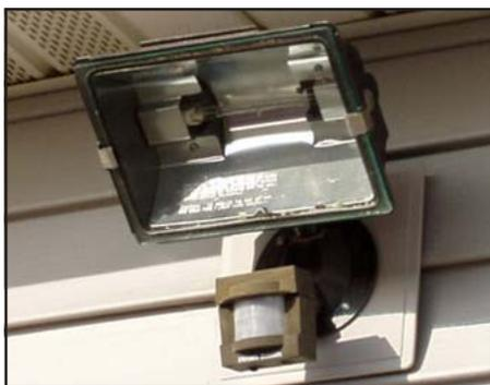
**Figure 7. Halogen yard light with a motion detector.**
